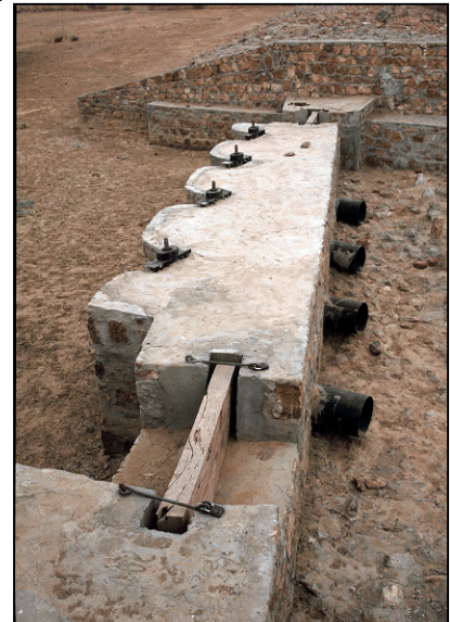
Earth Dam - Darfur
